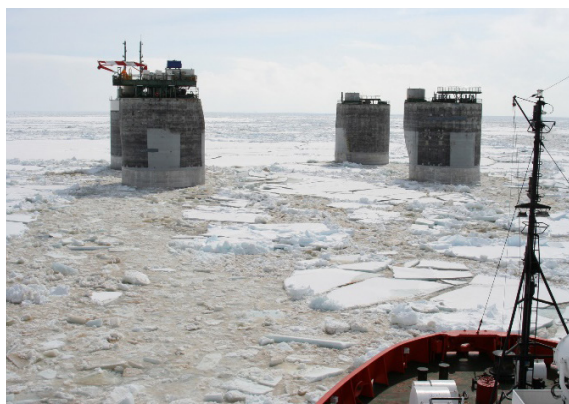
Fig. 11. Continuous first-year ice on phase III near the base of the MISP PA-B. Snapshot from a ship 04.04.2001.
